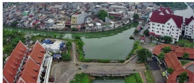
Figure 20. The Result of the East Canal Waterfront Area Source: PT Kind Indonesia (2023)
