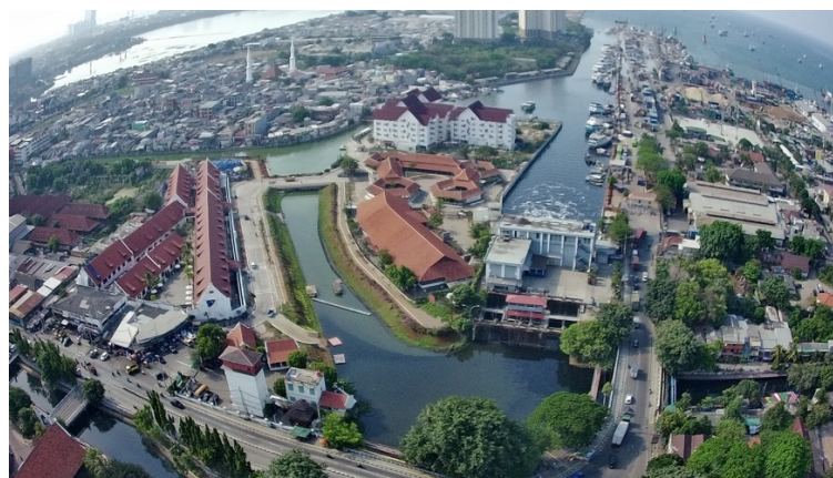
Figure 14. The Result of Bahari Diversion Channel – Aerial View Source: PT Kind Indonesia (2023)
