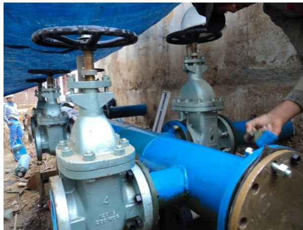
Figure 7. Gasket Inspection on Pipe Connection
